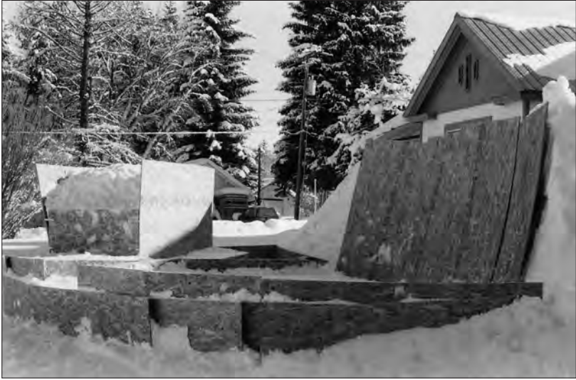
Fig. 24. Plywood forms help teams build up the base for snow sculptures.
